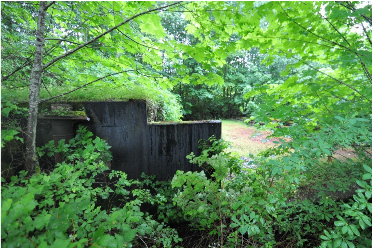
6. Old concrete farm building on subject in vicinity of home
