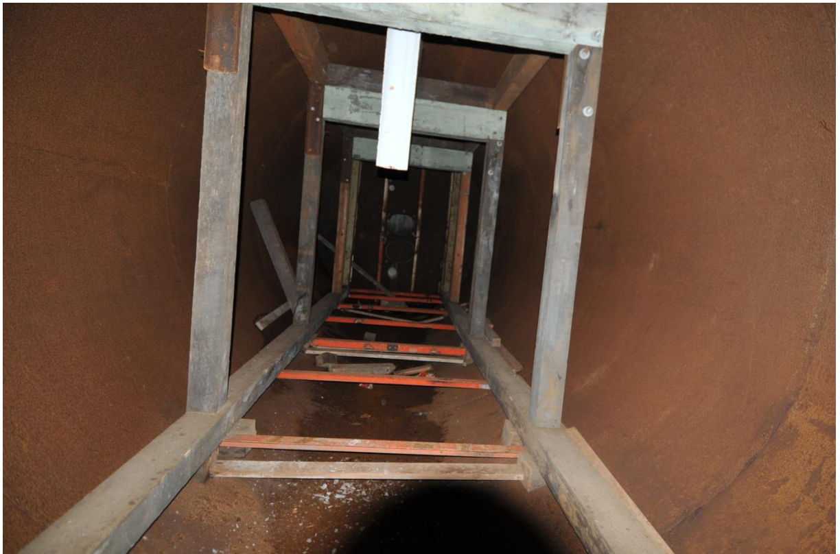
8. Interior view of bomb shelter, located in the rear of the concrete structure
