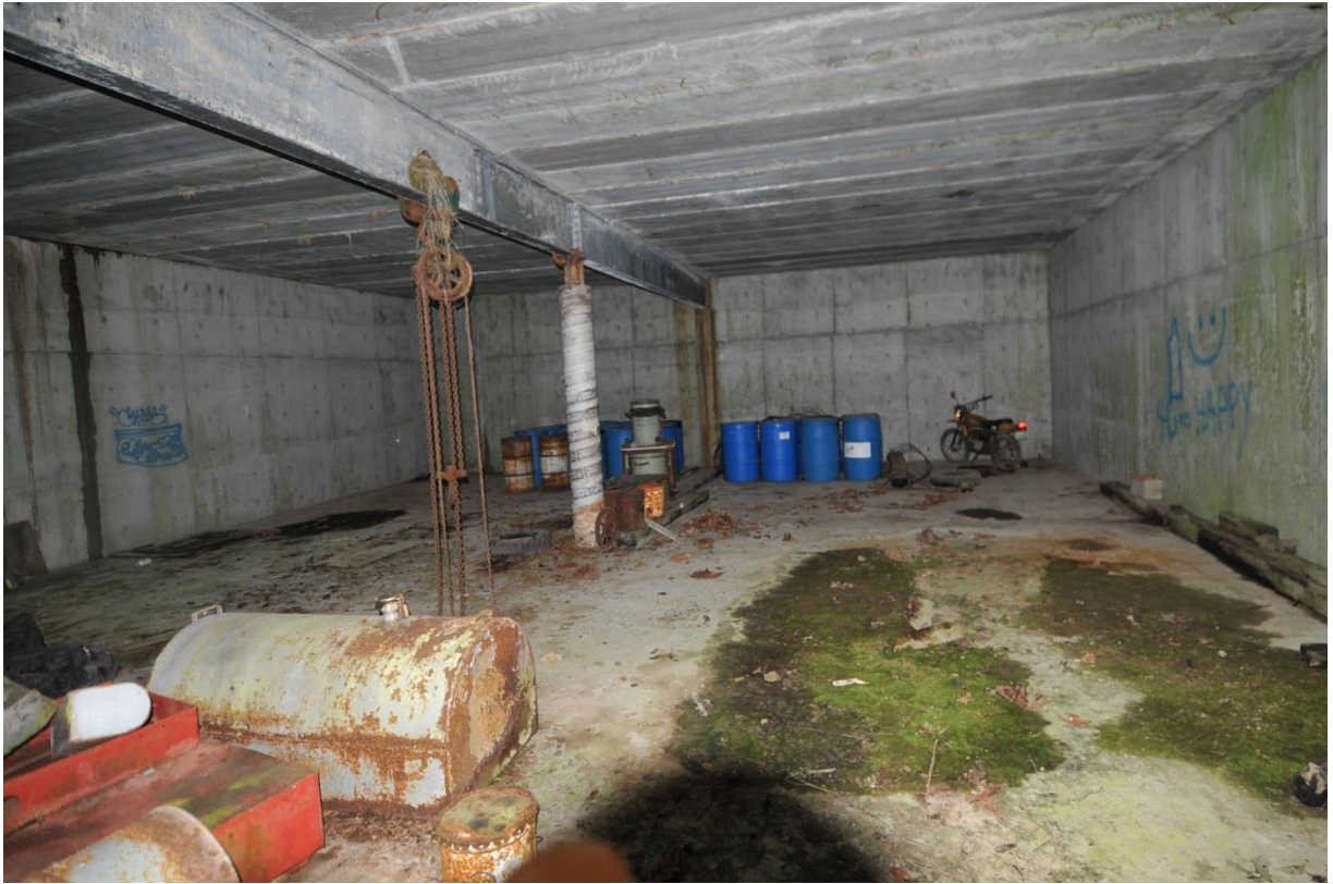
7. Interior view of structure old concrete farm structure on subject in vicinity of home
