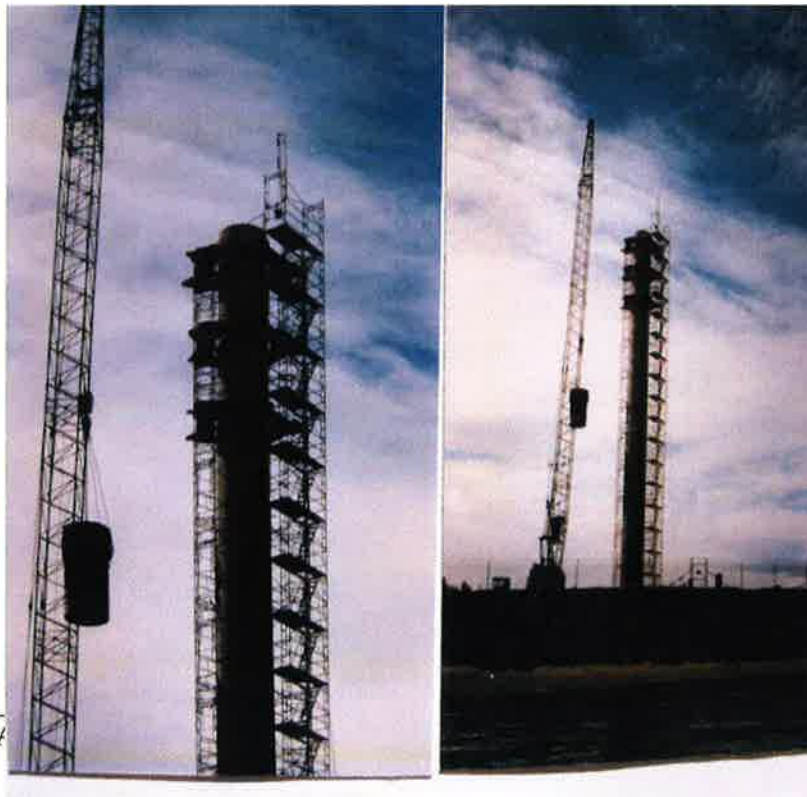
Figure C-8 Removal of the Smokestack
