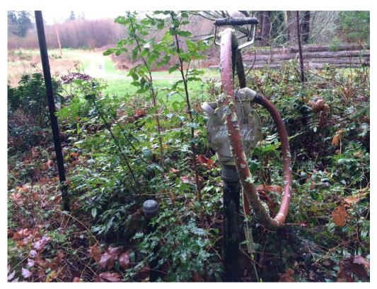
Photograph 4. Pump for Petroleum UST
