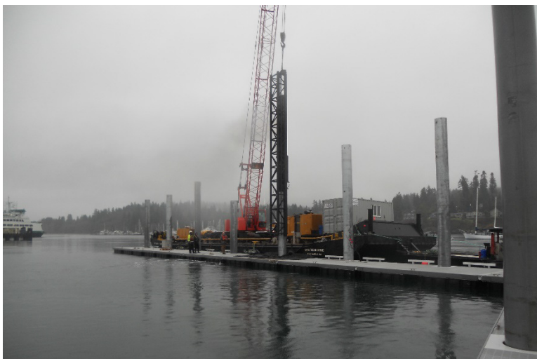
Figure 10. Barge crane installing piles at City Dock
