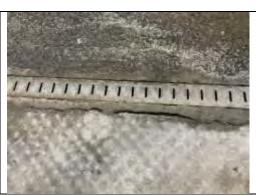
4. Corrosion and scaling at south end steps
