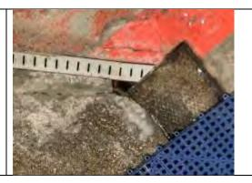
3. Deterioration at trench drain <u>The linear trench drain</u> <u>extends around the entire pool. The drain is reportedly</u> working as intended.
