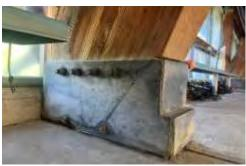
9. Glu-lam beam and wood decking roof faming <u>Findings:</u> <u>Glulam wood arch beams and timber T&G</u> <u>decking support the semi-arched clear-span over the natatorium.</u> Where the framing was observed up close and soundings made, the glulam beams were found to be in good condition with no signs of deterioration or structural cracking at the laminations.
